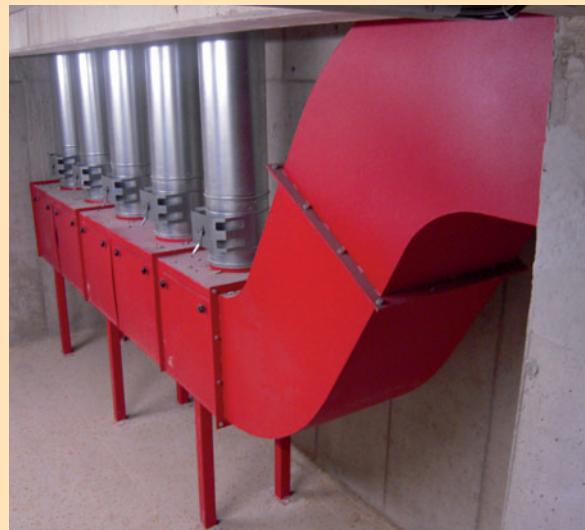
Usage of existing warm air from other parts of the plant
